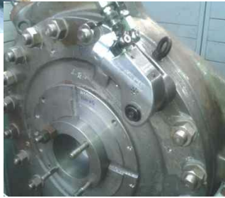
◀ PSD-3 Bolt tightening of Centrifugal pump casing
